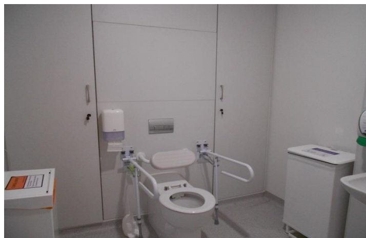
Picture 1: Newly Refurbished Patient Toilet
