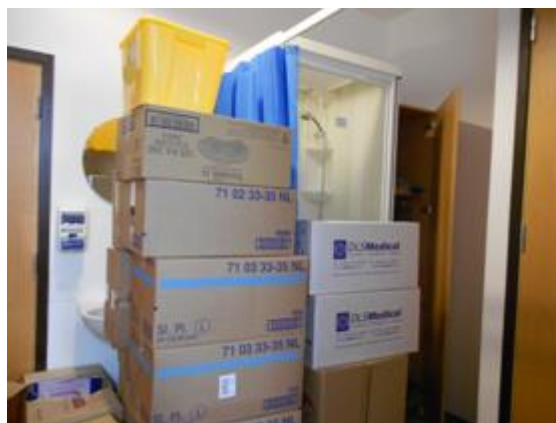
Picture 2: Side room used as a store. Cluttered room and stock blocking access to shower cubicle.
