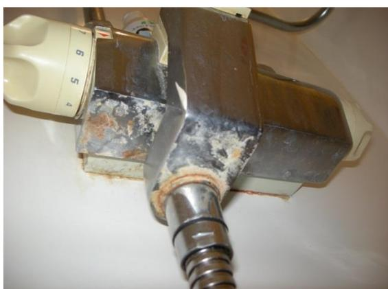
Picture 1 – Underside of shower fixture
