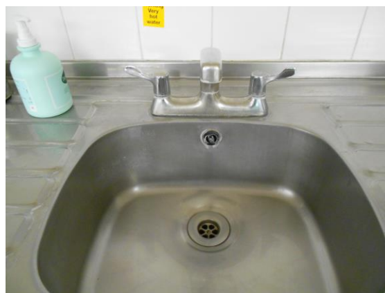
Picture 5: Hand washing sink with overflow and small twist taps at the nurses' station in M1
