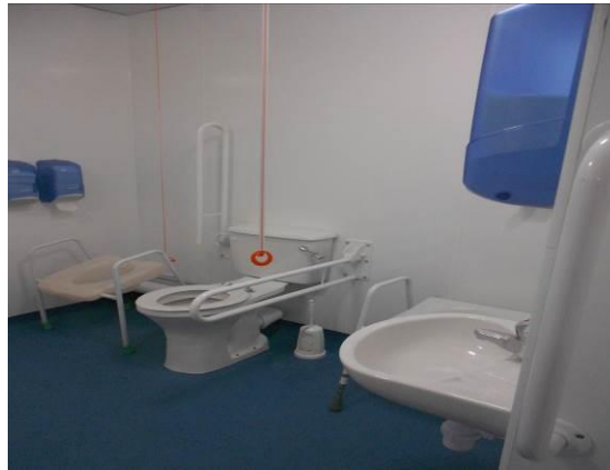
Picture 3: 6N Refurbished sanitary facility
